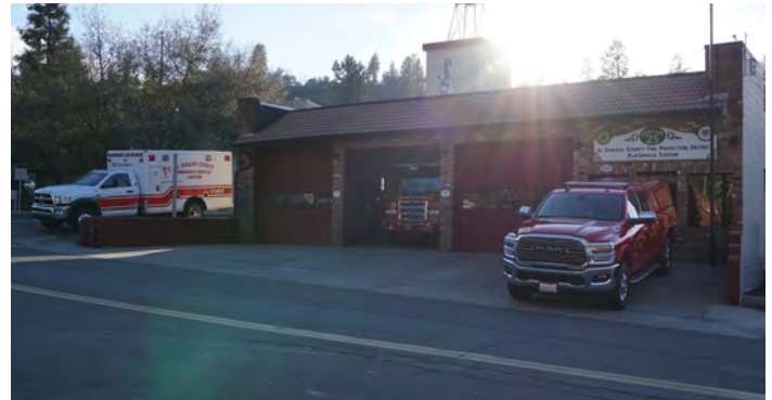
View of Station 25 from Sacramento Street
