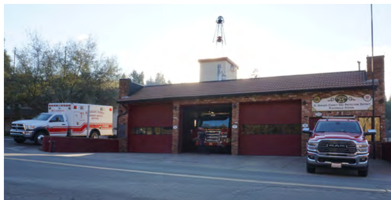
CITY OF PLACERVILLE Station 25
